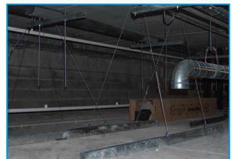
Under panel evaporator
