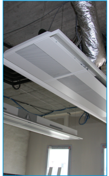
Chilled beams
