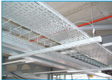
Multiple cable trays on single channel
