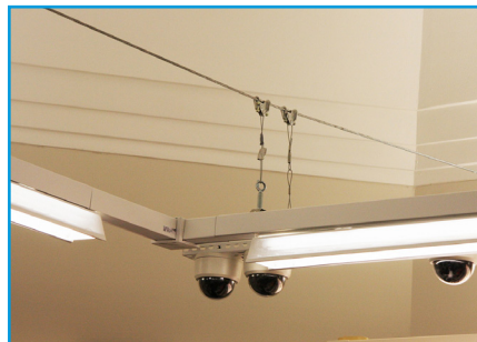
Lighting and Camera on Catenary
