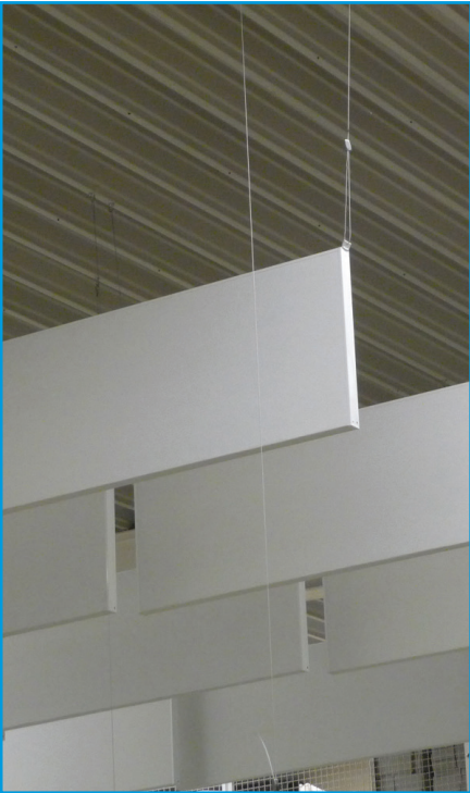
Acoustic baffles
