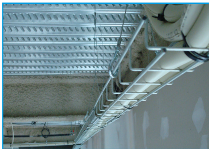
Refrigerant pipes
