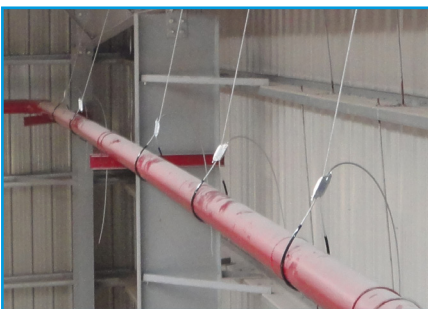
Intermediary supports for steel pipes
