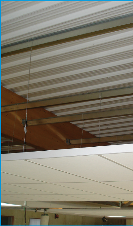
Suspended raft ceilings
