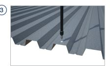
Drill the hole for the Spider Metal Deck.
