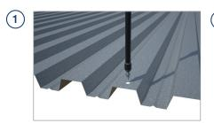
Fit the Spider Stepped Drill Bit to the Spider Drill Chuck Extender. Then attach to a drill and drill holes into the metal deck.
