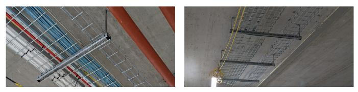
"On this job we were putting different sizes of cable baskets onto the Fast Trak brackets. Thankfully Gripple's Fast Trak brackets come pre-cut to certain lengths and Gripple's drawings were all set up for us. The brackets and baskets fit together seamlessly and their Cable Basket Clips simply twist in by hand, making the speed of installation brilliant!"
